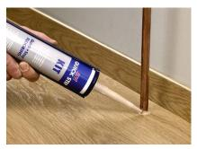
Apply the kit to the joints with the aid of a Sealant gun. Cut the plastic spout off at an oblique angle, making an opening of at least 5mm/0.2 In diameter. Then apply the kit to the joint and spread it smooth with a filling-knife. The joints must be clean, dry, dust and grease-free.
